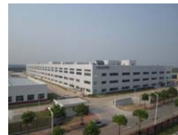
New factory in Guangzhou, China
